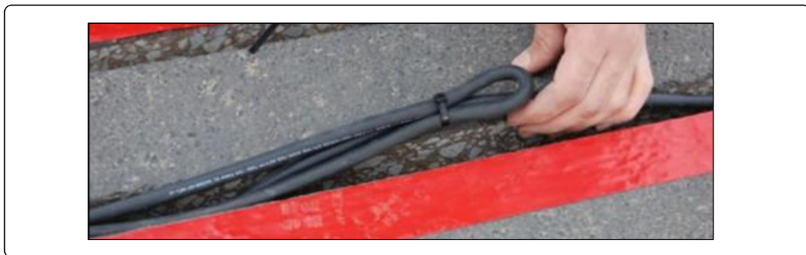
Figure 7-C: Tying Cables with Zip Ties
